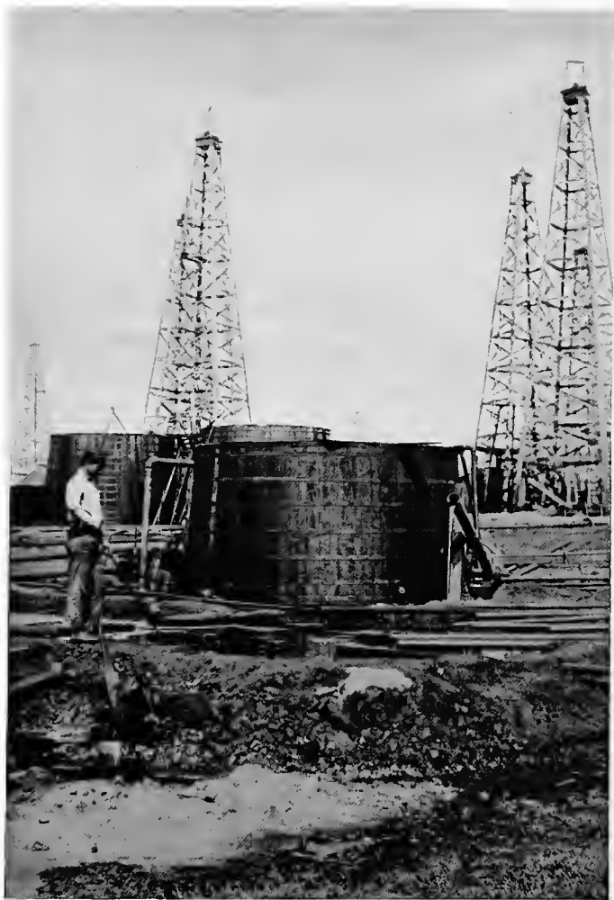
Some of the tanks among the derricks
